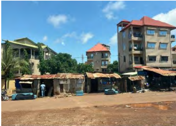
Figure 13-14: Views of housings along RO308 (to the east)
