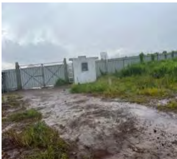
Figure 13-4: Site fence and security gate
