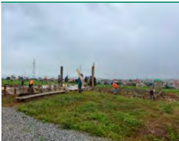
Figure 13-6: ACC's welfare facility area
