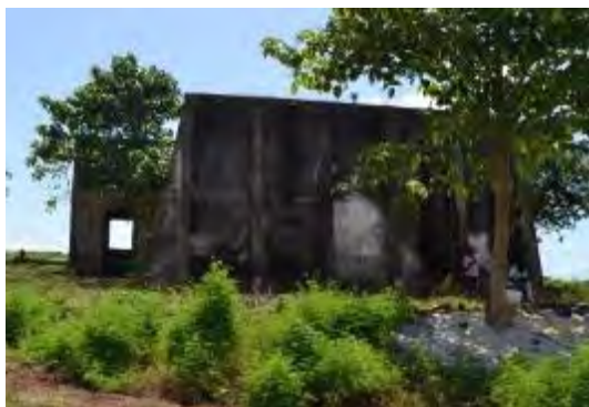
Figure 13-19: SEG Water Pumping Station and Water Tank (view from outside) adjacent to the Project site
